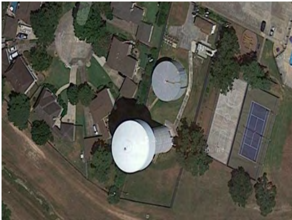
Water Plant Site Overall
