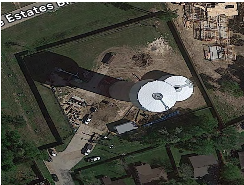
Water plant site overall
